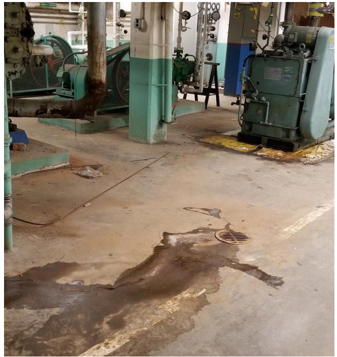
Stained Floor Drain
