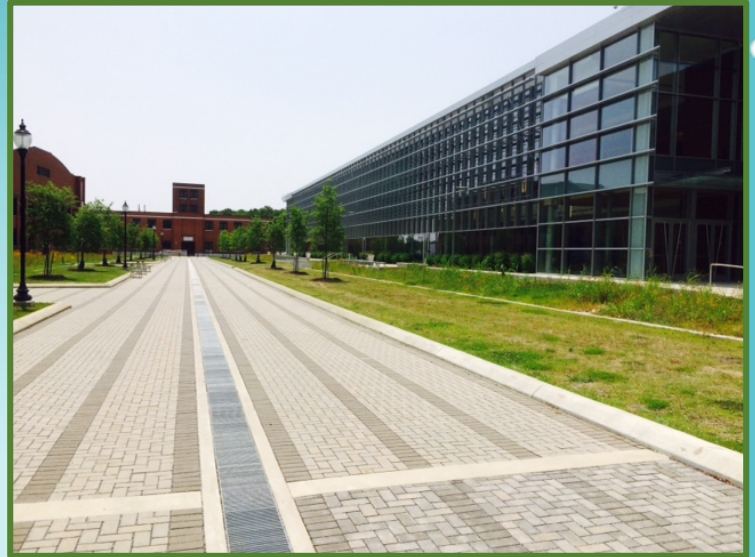
Permeable pavers installed along IESB (B2102) at LaRC.
