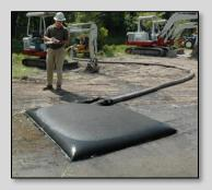
For construction-related dewatering operations, the contractor must dewater in accordance with a plan approved by the Environmental Office. Typically, the contractor will use a dewatering bag or similar BMP for this type of action.
