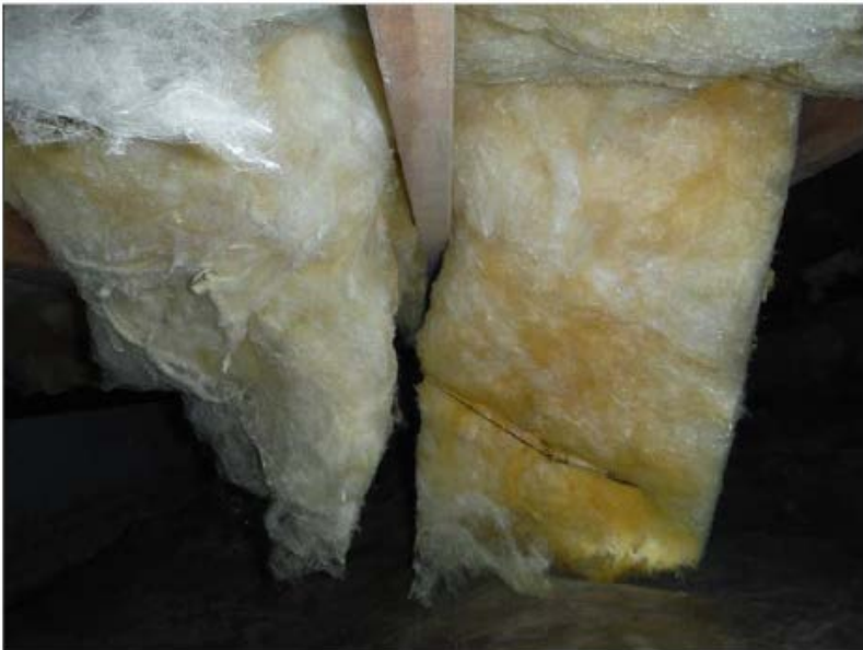
8.5 INSULATION Picture 1 Typical Loose Insulation
