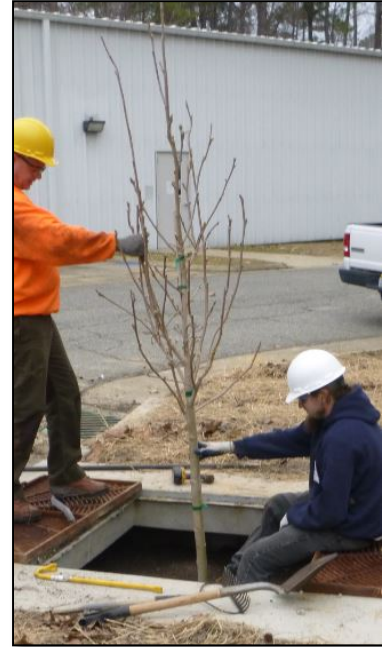
CONTRACTORS INSTALL A TREE BOX FILTER
