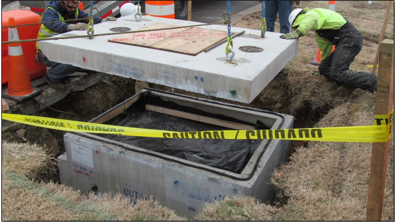
CONTRACTORS INSTALL A TREE BOX FILTER
