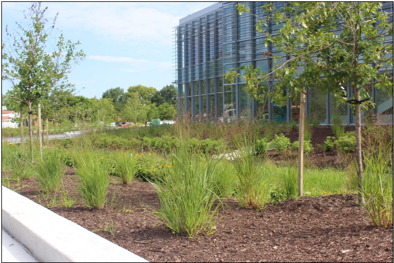
BIORETENTION AREA AT IESB, BUILDING 2102
